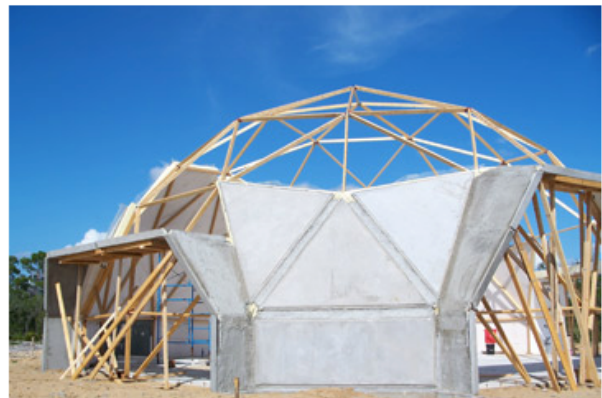
Dome homes may have nontraditional designs, but they can still incorporate traditional construction materials, such as wood beams and concrete.
