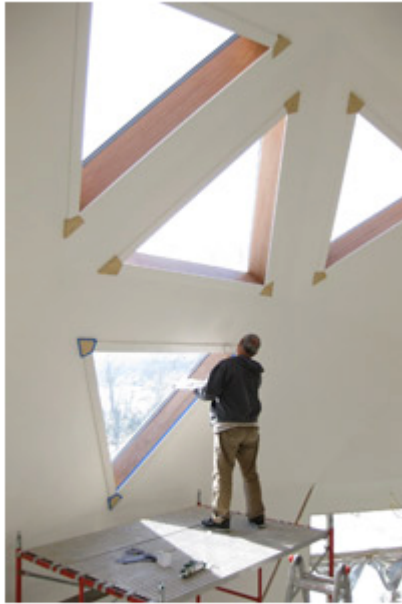
The triangular windows of this home serve as a reminder of the geometric shape that helps make this dome structure so strong. Image courtesy Timberline Geodesics
